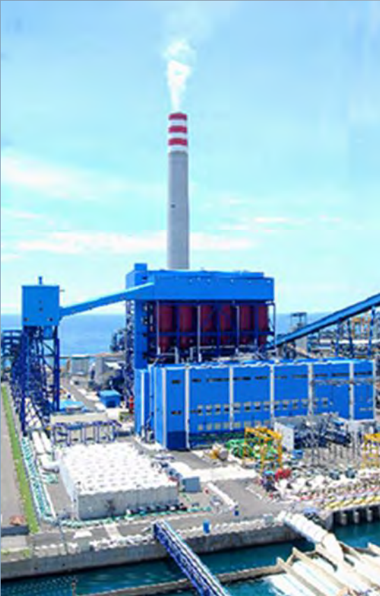
Paiton Private Power Project in Indonesia
